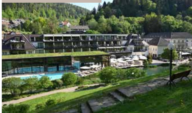
HOTEL THERME BAD TEINACH
